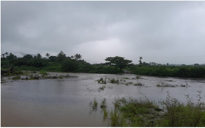
Figure 12g: Toge Crossing (Nacaci) in Ba underwater on the 22 nd . Source: Fiji Roads Authority.
