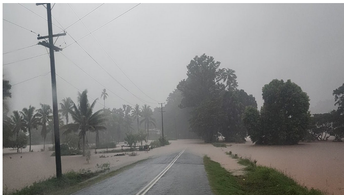
Figure 12a: Bulileka Road at Urata/Boca Junction on the 12 th . Source: Fiji Roads Authority.
