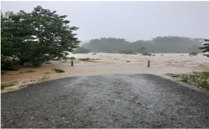
Figure 12i: Waima bridge underwater in Naitasiri on the 24 th . Source: Fiji Roads Authority.
