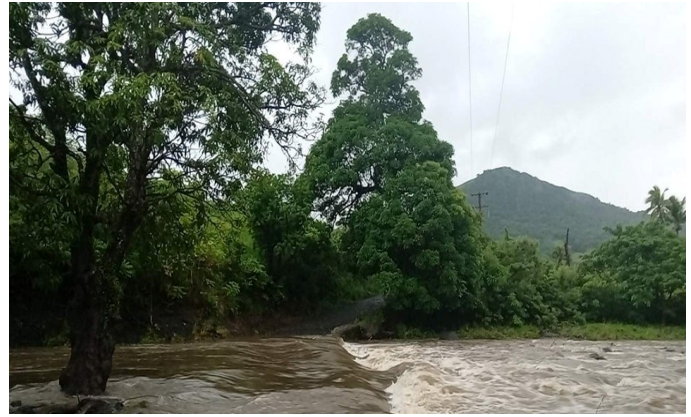
Figure 12h: Narara Road, Rakiraki on the 22 nd . Source: Fiji Roads Authority.
